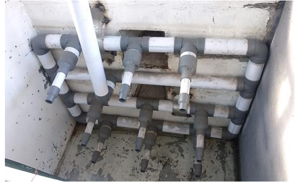
Gambar 9. Nosel berbahan Pipa PVC
